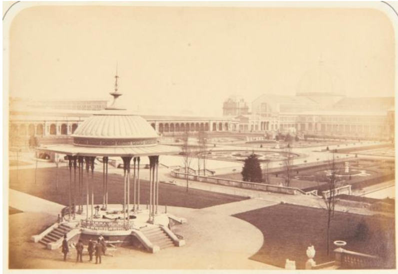
Figure 2: Charles Thurston Thompson, Horticultural Gardens, South Kensington, 1862 , showing the 'band house' under construction. Albumen print, 13.4 × 19.6 cm (Royal Collection Trust; © Her Majesty Queen Elizabeth II 2020 < http://www.rct.uk/collection/RCIN_2932800 >)
